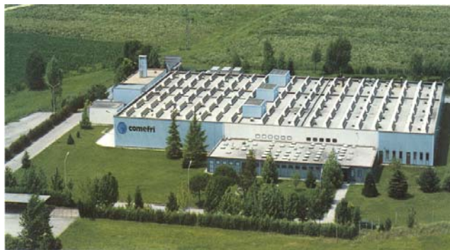
COMEFRI SpA factory at Arterga (UD) – Italy with 6.300 m 2 workshop. Production of industrial fans and special executions. Test facilities: laboratory accredited by AMCA and SINAL.
