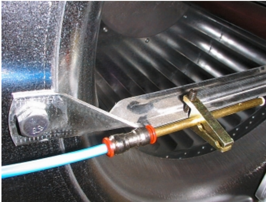
Figure 3: Installation of sensor
